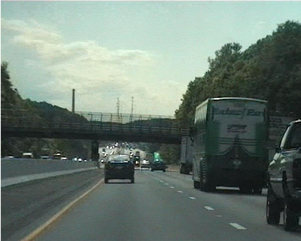
Image after deinterlacing
